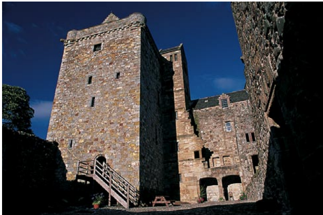
The tower with an original entrance in the west wall, the new stair turret and the east range with ground floor loggia (open arcade) © Clackmannanshire Council
